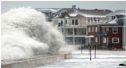
Coastal flooding Spring tides and storm surge
